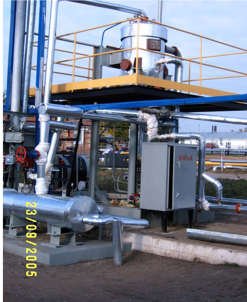
REACTOR WITH FLUIDIZED BED OF GRANULATED CATALYST (BAVLY CRUD DEPOSIT AT REPUBLIC OF TATARSTAN)
